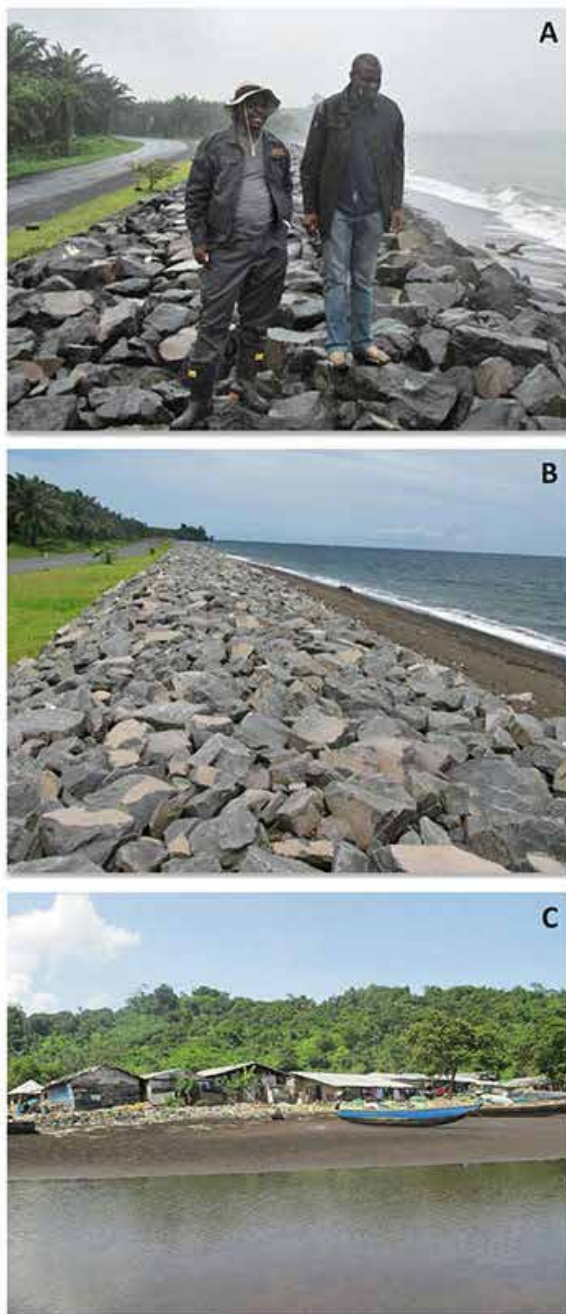
FIGURE 3. Coastal settlements (A) and road infrastructure (B&C) threatened by storm surges and sea-level rise with an embankment constructed to protect the road at Debunscha, Fako Division, South West Region, Cameroon. (Photo credit: Prof. Samuel Ndonwi Ayonghe)
